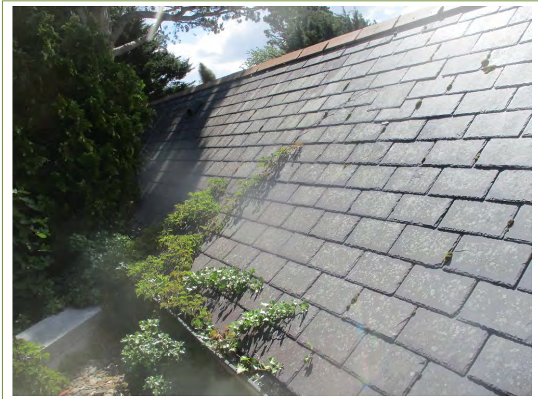
Natural slates on the roof of the swimming pool
