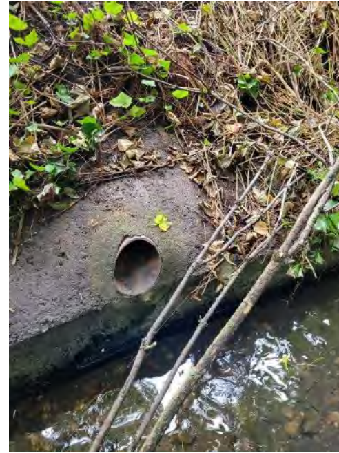
Figure D Site 1 - Storm drain
