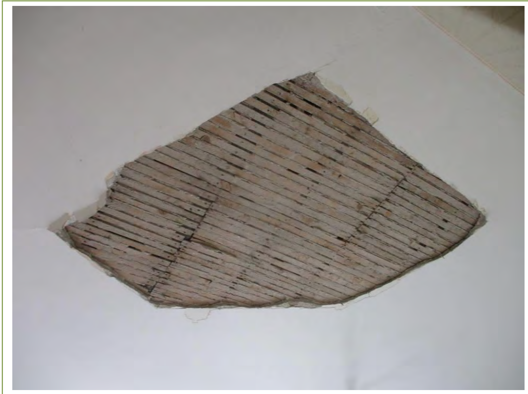
Lath and mortar ceilings in the main house
