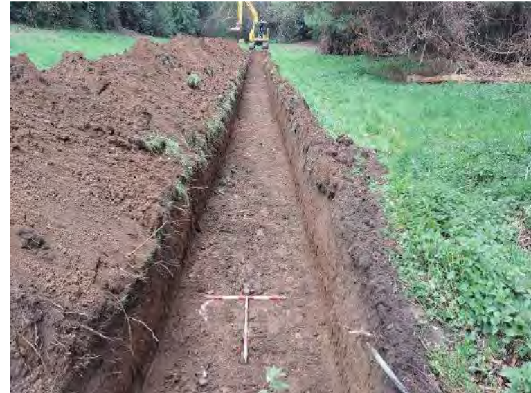
Plate 6 –Trench 1, facing northwest
