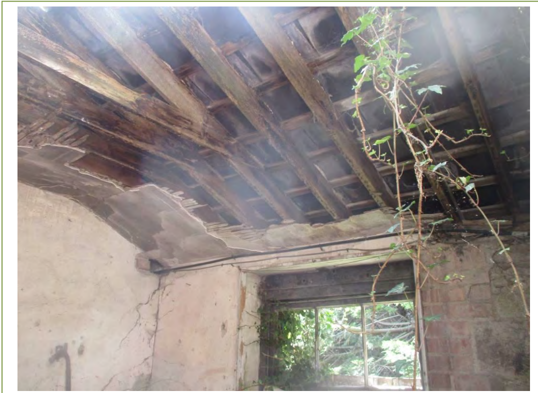
Natural slates on the roof of the rear derelict buildings
