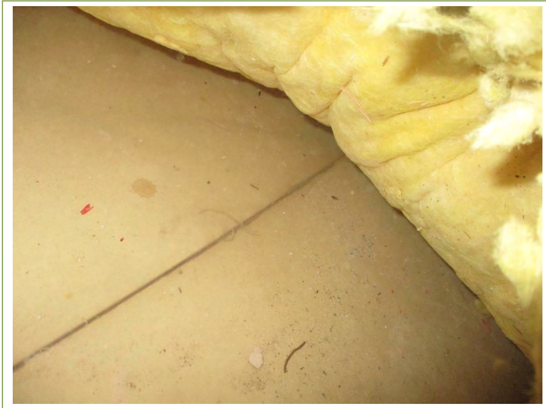
Plasterboard and fibre glass insulation in the occupied gate lodge
