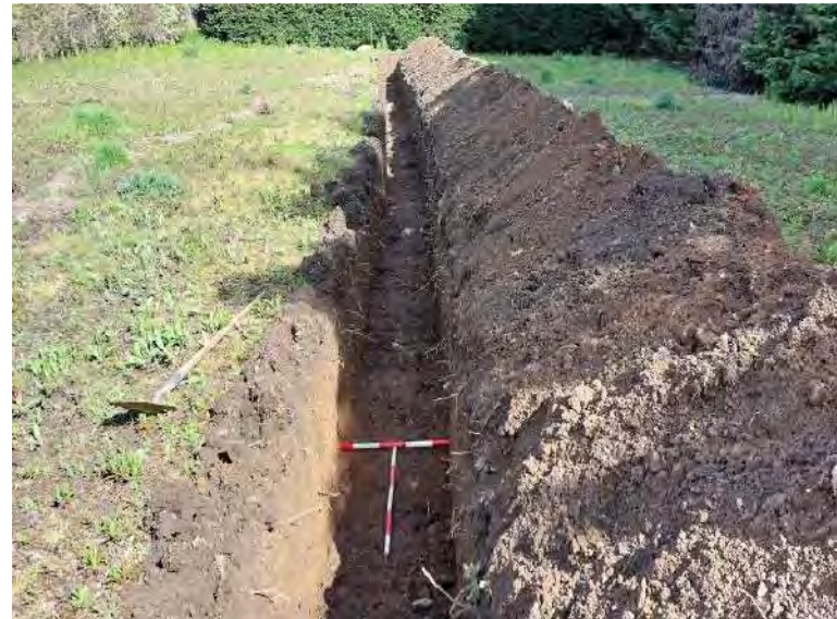
Plate 12 – Trench 16, facing north
