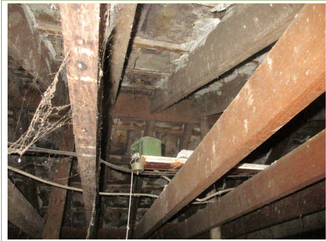
Slates on the main roof
