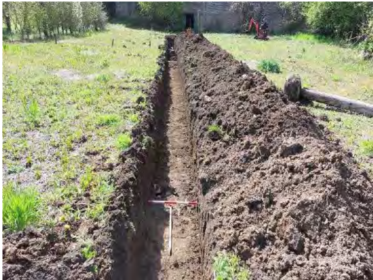
Plate 11 – Trench 15, facing south
