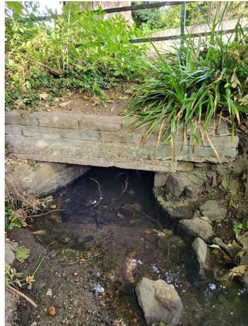
Figure F Site 2 - Facing downstream
